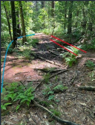
Approach view — old pallet bridge & wetland crossing
